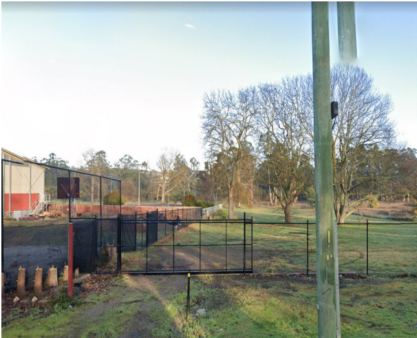
Picture 7 – Southern Interface to No.363 Swansea Road
