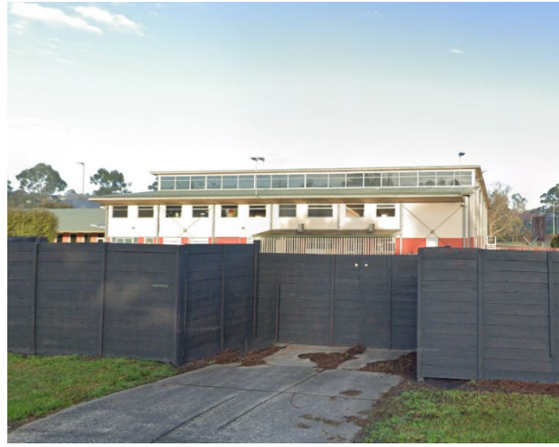
Picture 8 – Existing buildings at No.363 Swansea Road
